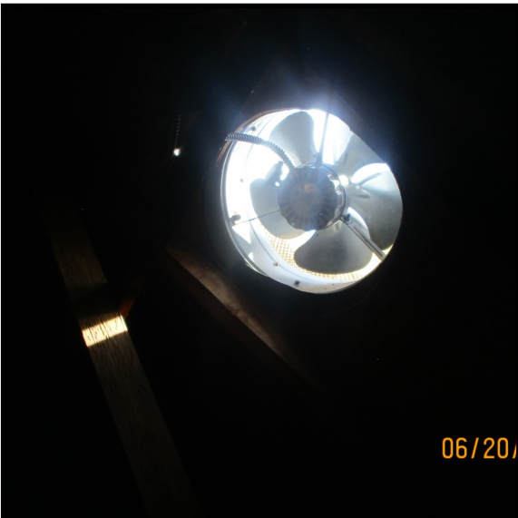
Roof fan in the attic
