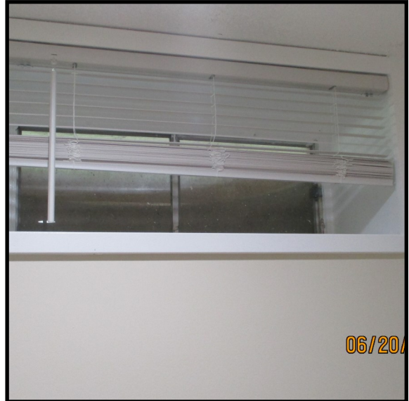
Windows in the basement
