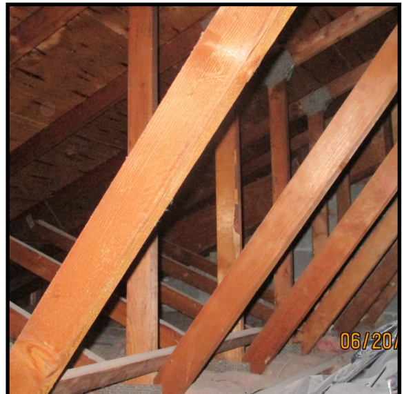
View of roof rafters in attic
