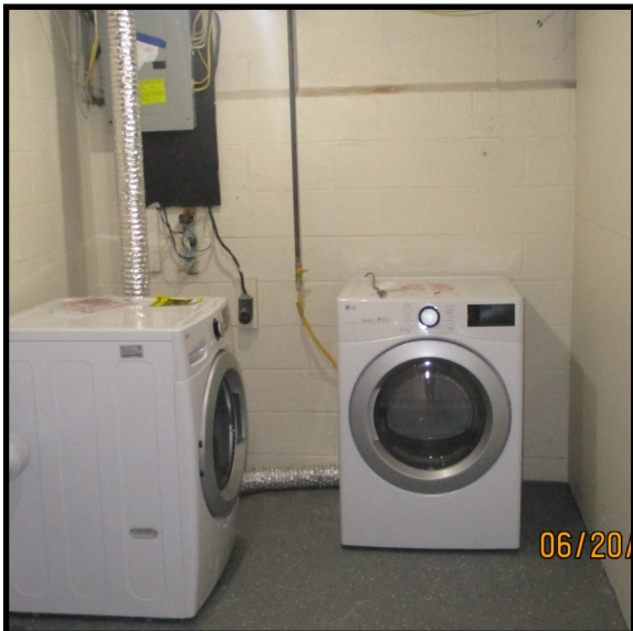
View of laundry room
