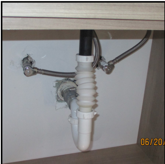
P-Trap underneath sink in 1st bathroom
