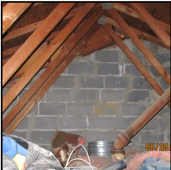
View of attic
