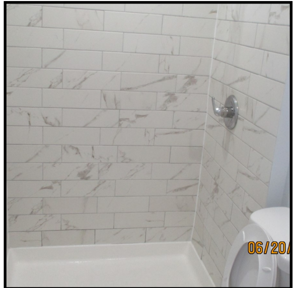
View of shower in bathroom
