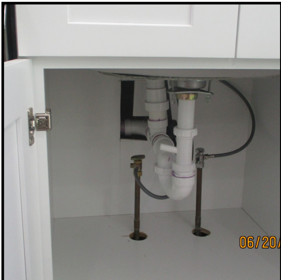
Underneath kitchen sink
