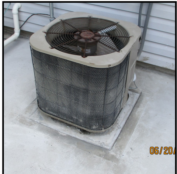
Old AC unit at the back of the house
